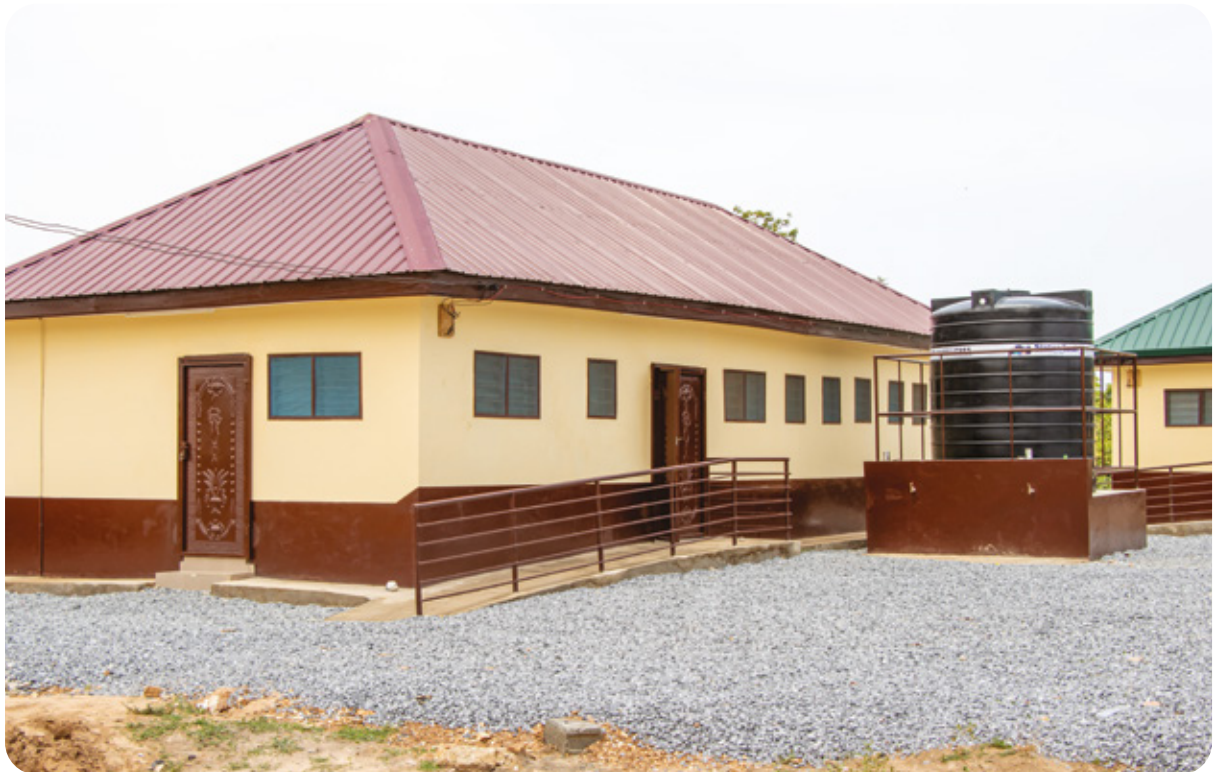
A typical GAMA SWP Modern School Toilet.
