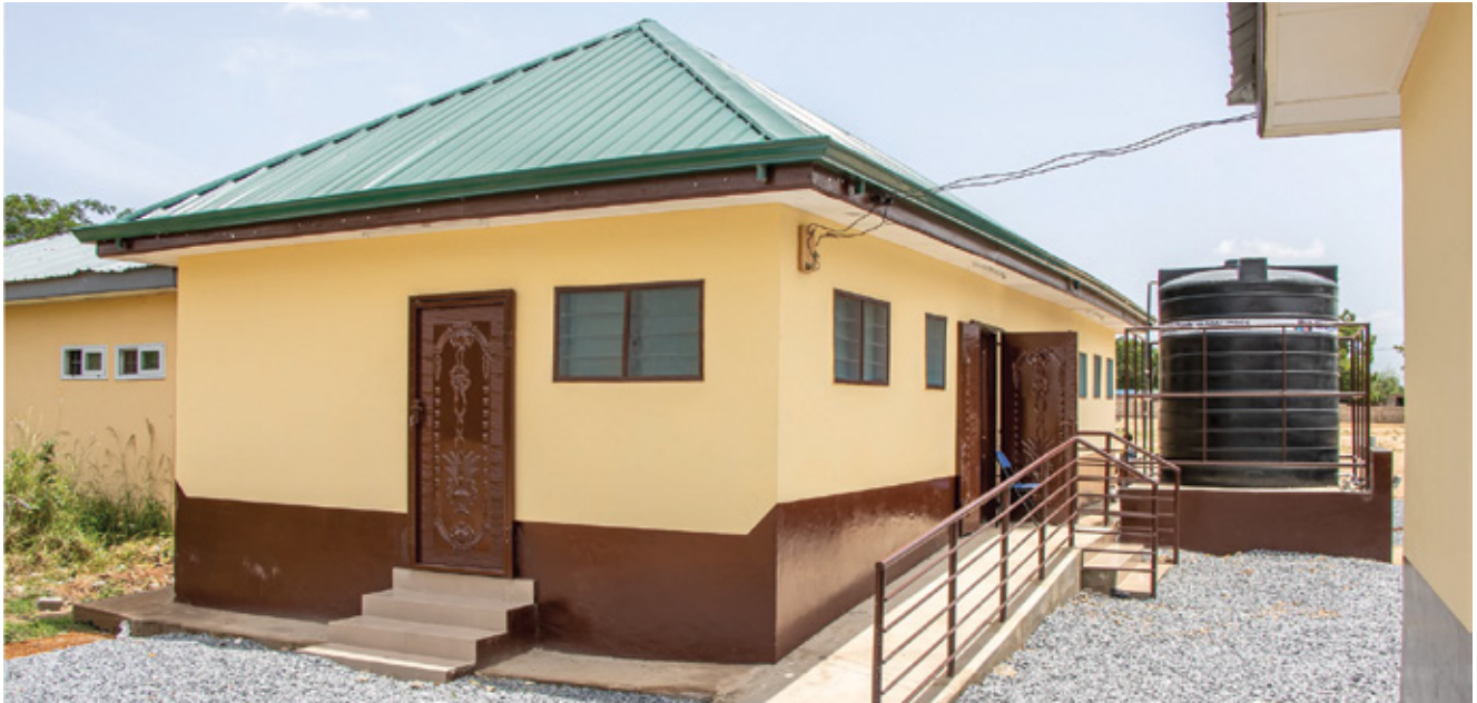
External view of a typical GAMA SWP school toilet facility
