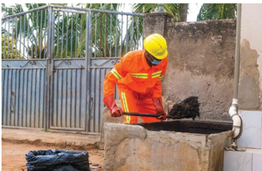
A professional bio-digester emptying activity
