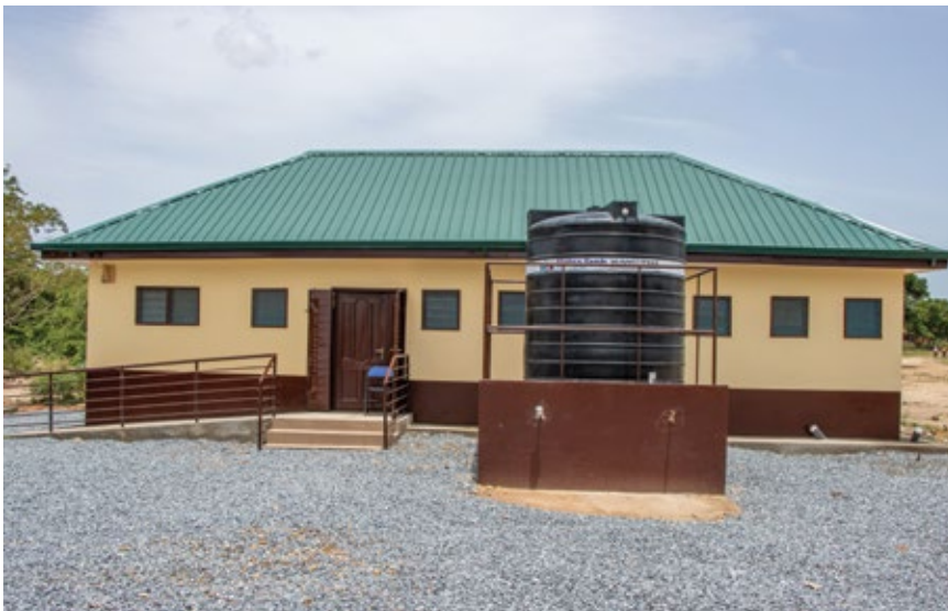
A completed GAMA SWP school toilet in Accra
