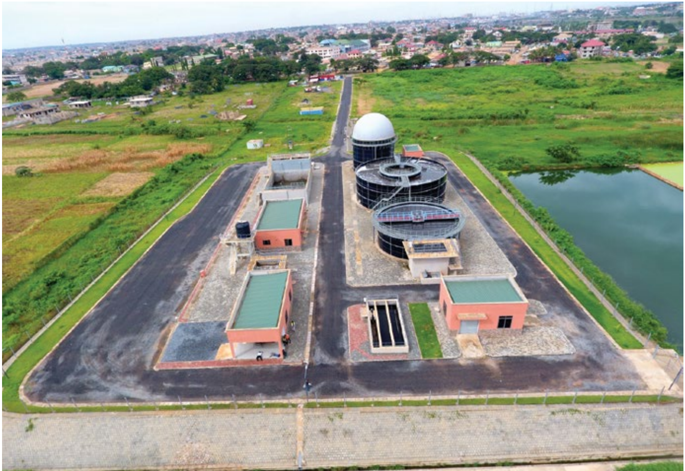
Aerial view of the Ashaiman Sewerage Treatment System
