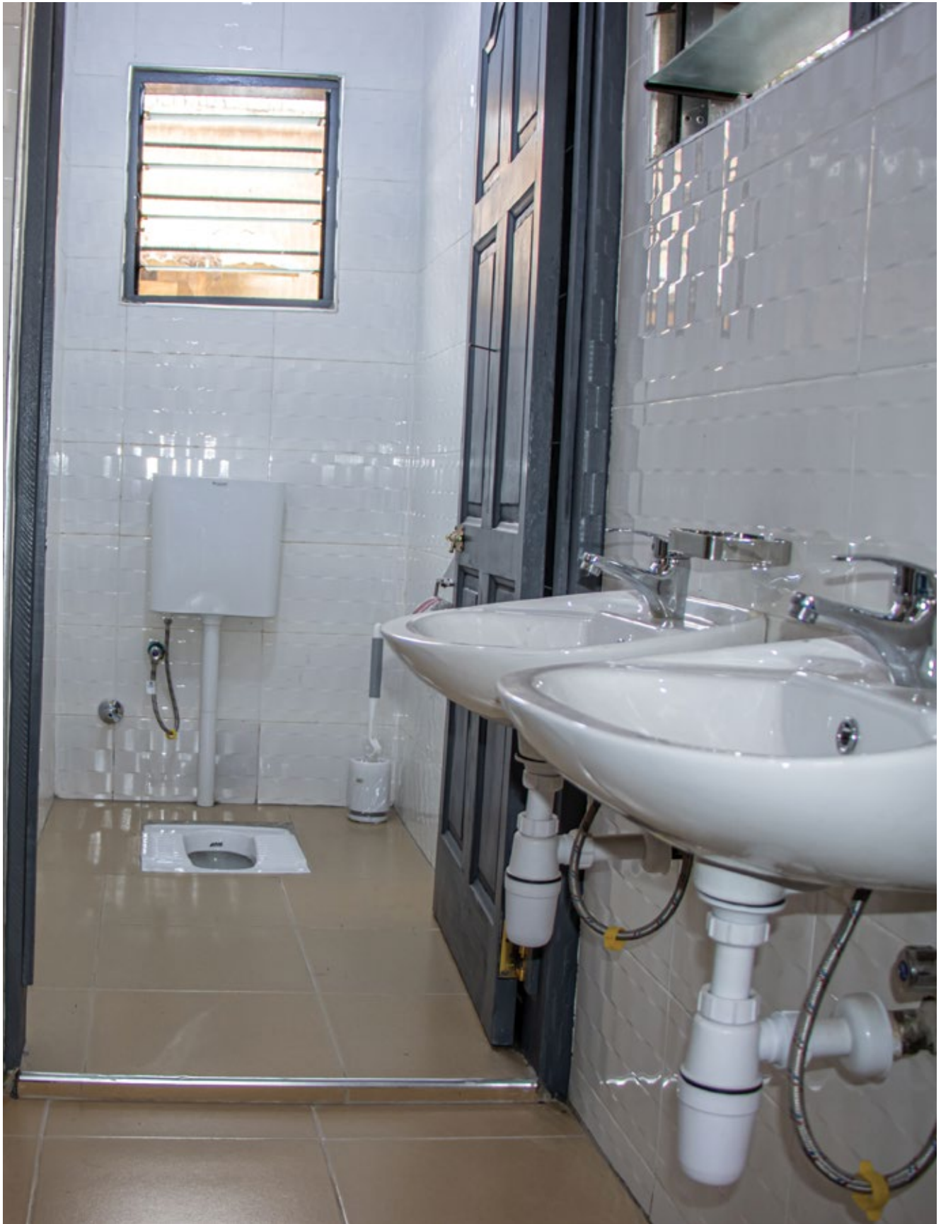
A well maintained school toilet facility
